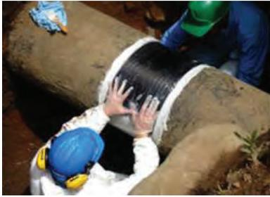
The structural system forms a pipe around a pipe, and each successive wrap increases the pressure rating. Its bidirectional weave allows for strength in both the hoop and axial directions experiencing little or no creep properties over time, ensuring that there is no reduction in strength.
